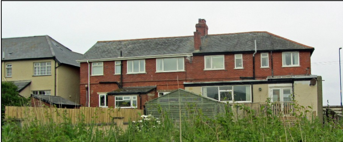
The rear of the pair of houses in 2016.
