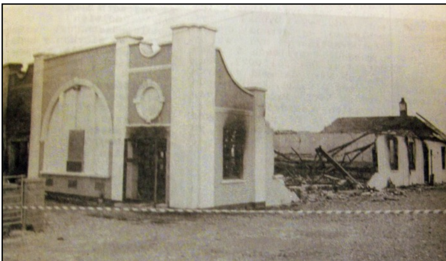
A photograph in Y Tincer of June 1993 taken by Anthony Pugh shows it after the fire. It had an important looking front built of brick, rendered, and with tall flat pale coloured columns enclosing a large arched front window, the arch with a keystone and stops, and the two
