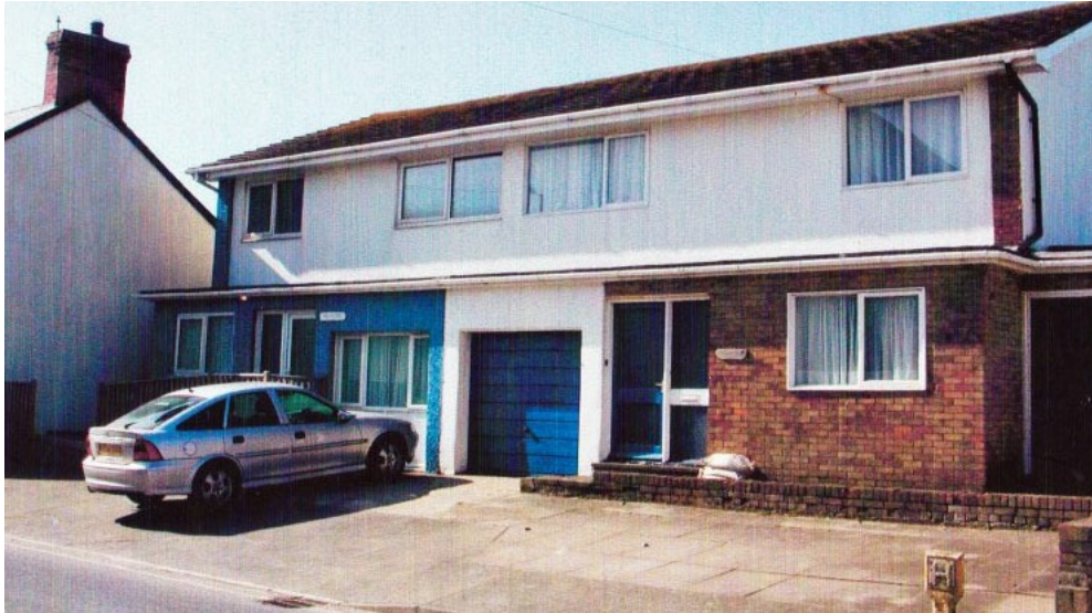
Water's Edge is the left hand house. This photograph was taken in 2009.
